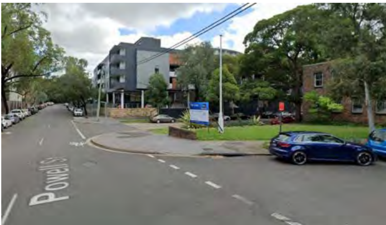
Photo 3: Powell Street looking west, with the apex of the site on the right, and sag point overflow point located at the end of the road. Source: Google Street View, dated March 2021.
